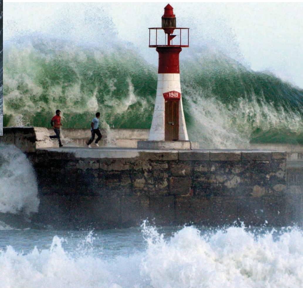
Need to build watch towers, dams, escape boats 12
